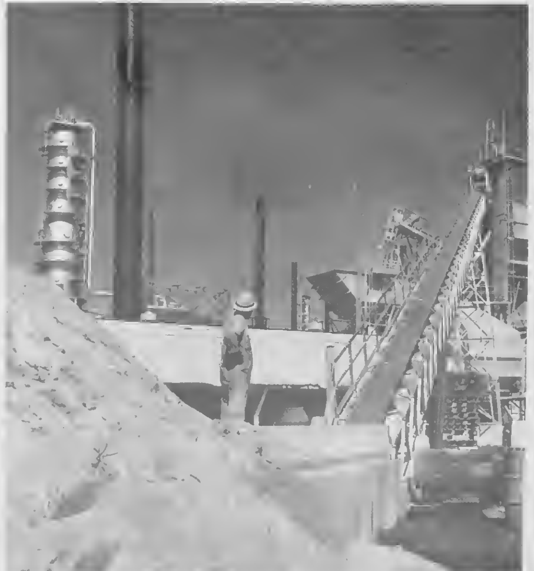
COPORAL DUNCAN watches a conveyor belt loaded with sand emerge from the tunnel and start its climb to the mixer.
